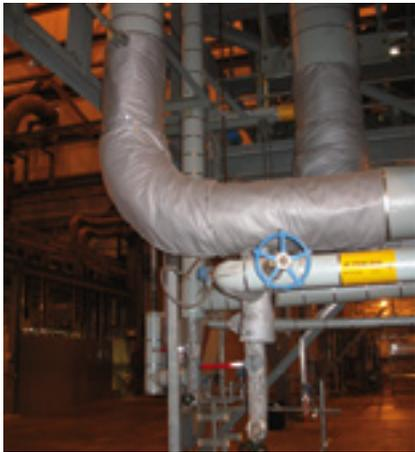
**3. Removable insulation** facilitates P91 hardness surveys
